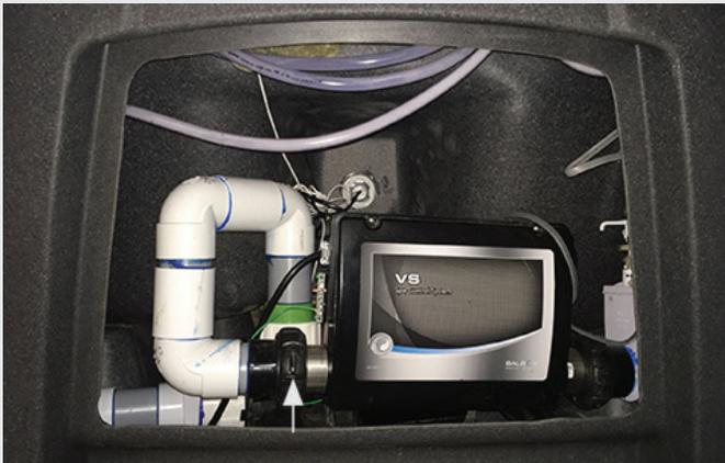
FIGURE 1.9a : HEATER UNION; LOOSEN UP TO BLEED AIR
