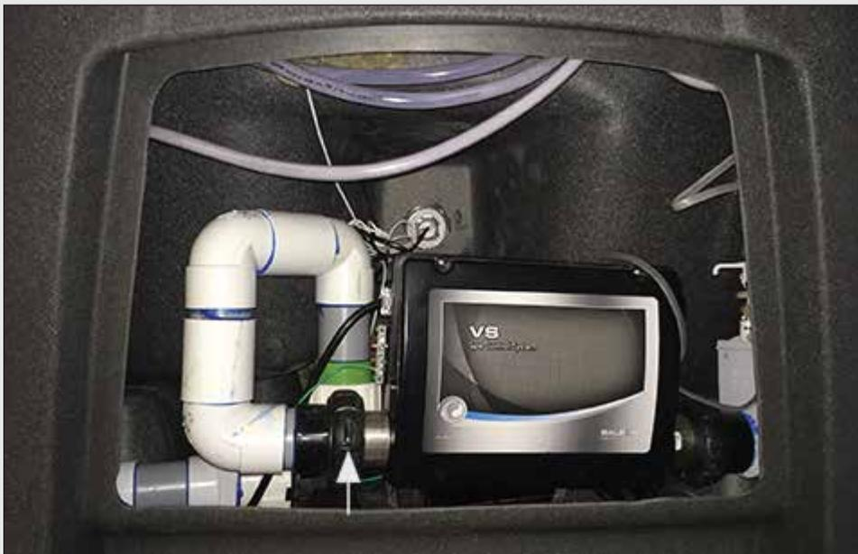
FIGURE 1.9 : HEATER UNION; LOOSEN UP TO BLEED AIR
